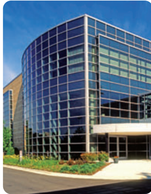
Offices | Lear Headquarters
