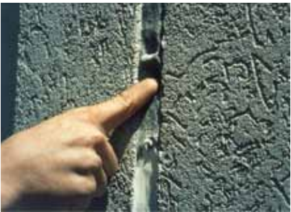
Polyurethane sealant cracking
