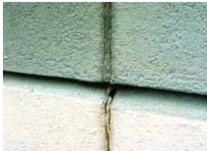
Polyurethane sealant alligating
