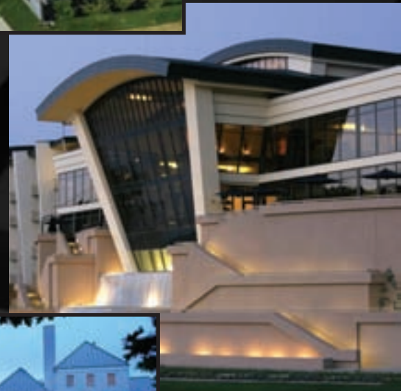
Inn of the Mountain Gods Mescalero, Mexico Architect: The Worth Group Award: Metal Architecture 2005 Design Award for Metal Roofing
