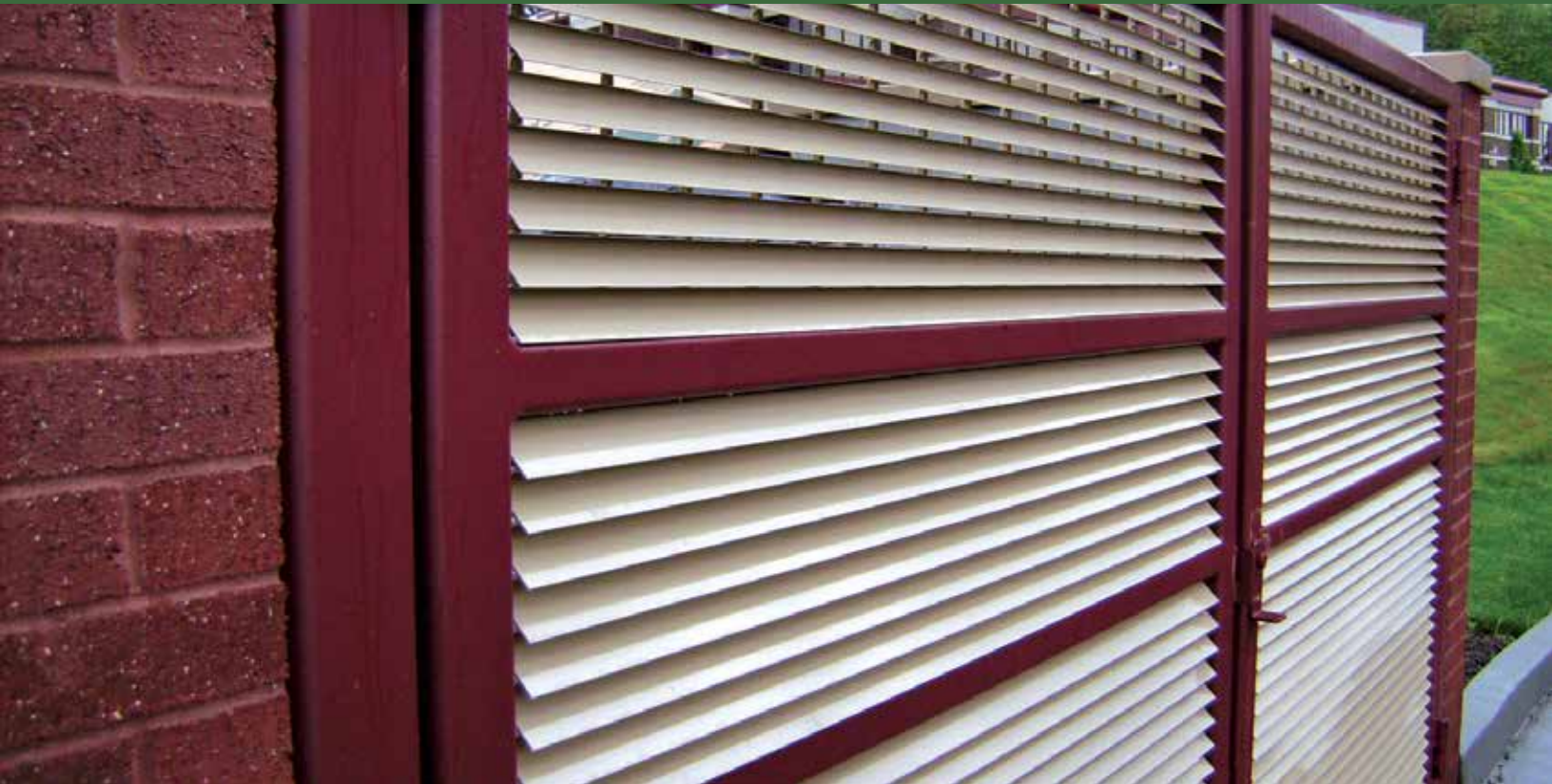
▲ Charles Pointe Office Building Bridgeport, WV LG80
