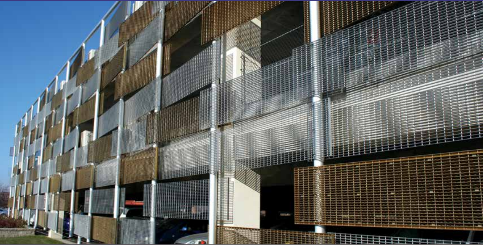
▲ Maplewood Mall Transit Center Parking Garage - St. Paul, MN 19SG4
