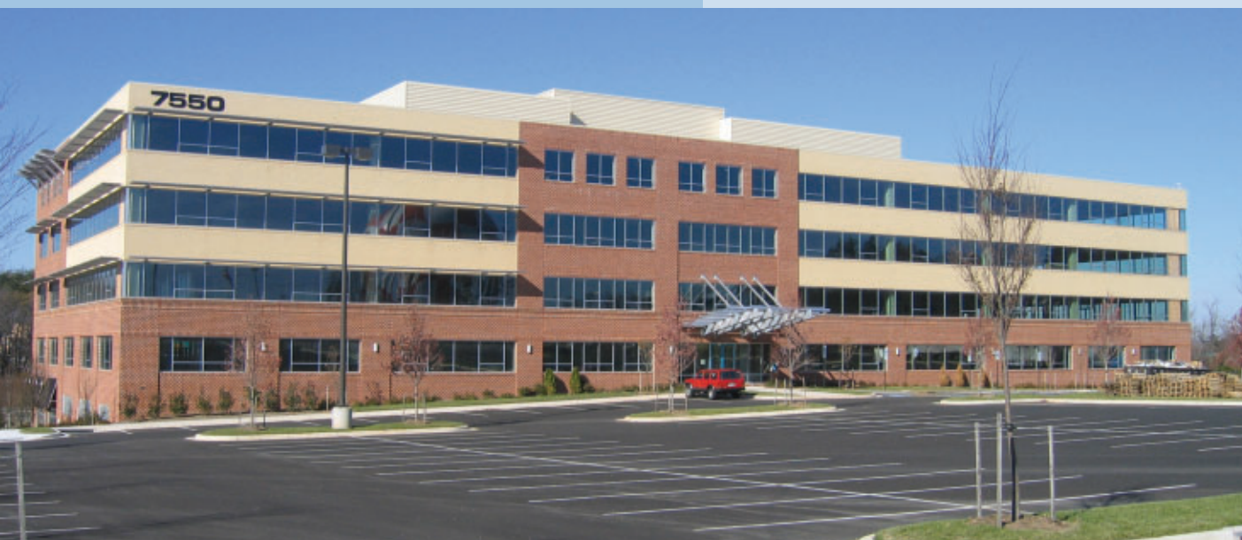
Developer/Multi-Tenant: Linden Associates, Arundel Mills Corporate Park, Hanover, MD, 110,000 ft 2
