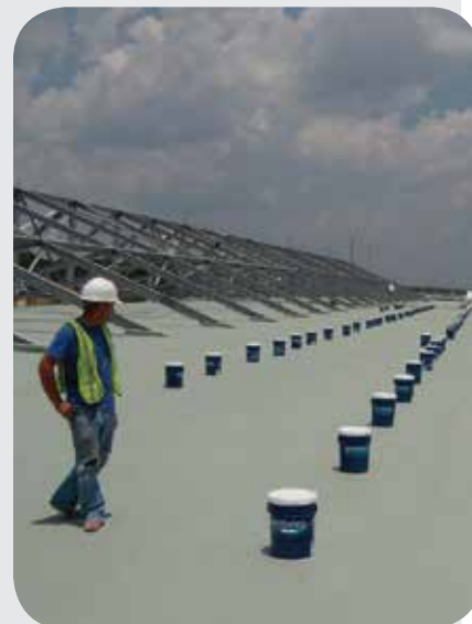
▲ National Guard Hangar - Jacksonville, FL
