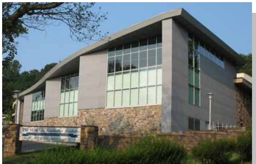
The Montclair Kimberly Academy, Montclair, NJ NK Architects
