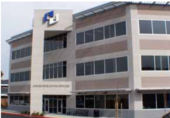
Harborstone Credit Union, Lakewood, WA The Casey Group Architects
