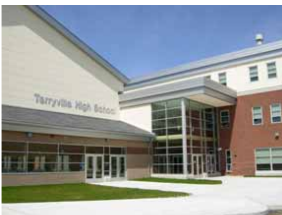
Terryville High School, Terryville, CT Jeter, Cook & Jepson Architects Inc.
