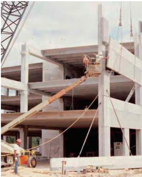
Figure 8-4 Spandrels being erected into pocketed columns.
