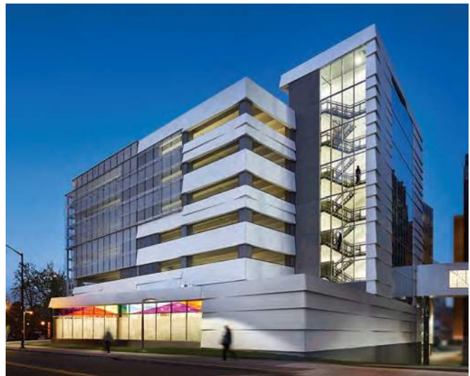
Figure 1-6. Hartford Hospital Hudson Street Employee Parking Garage - Hartford, CT (photo courtesy of Halkin Mason Photography)
