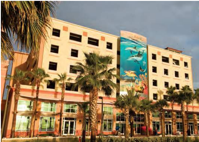
Figure 1-1. Surf Style Retail Store and Parking Structure - Tampa, FL (photo courtesy of Finrock Industries)
