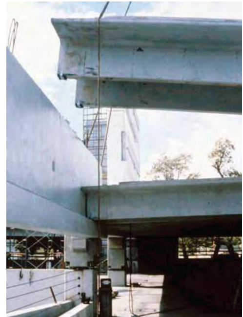
Figure 8-5 L-shaped spandrel being loaded with double tees.
