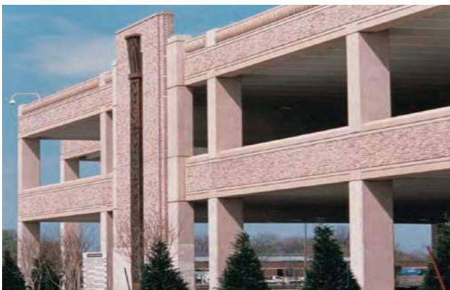
Figure 1-3. Shops at Willow Bend Parking Deck A – Plano, TX
