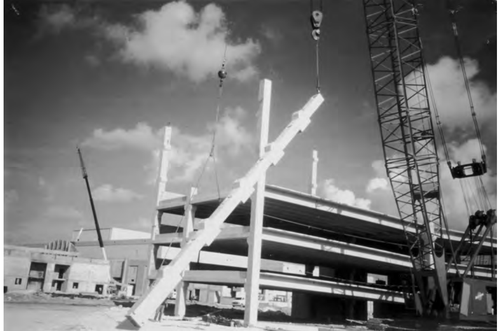
Figure 8-3 Rotating a column into position.
