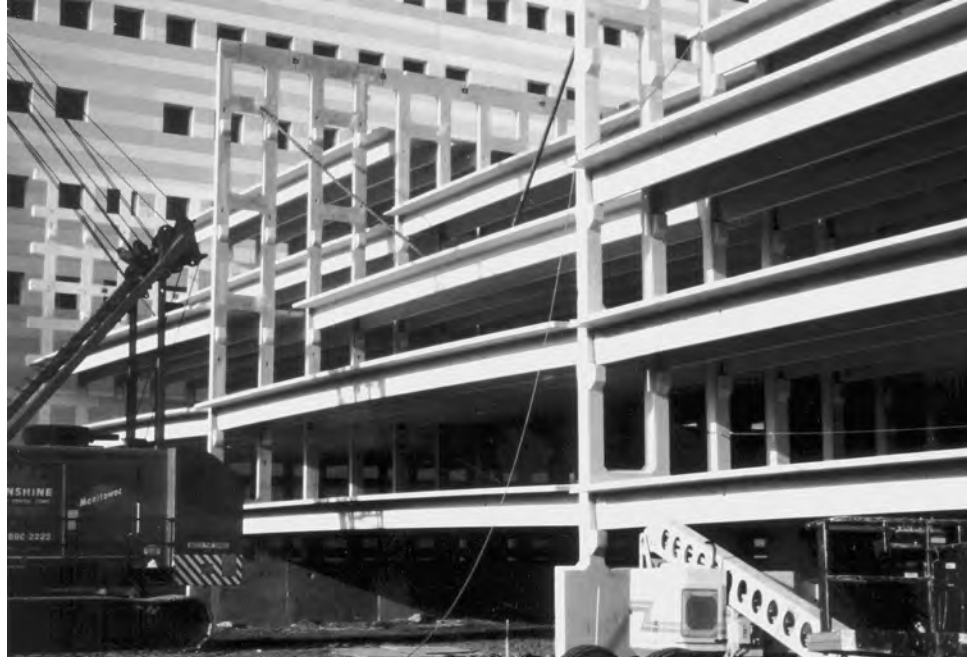
Figure 8-7 Braced litewalls during erection.
