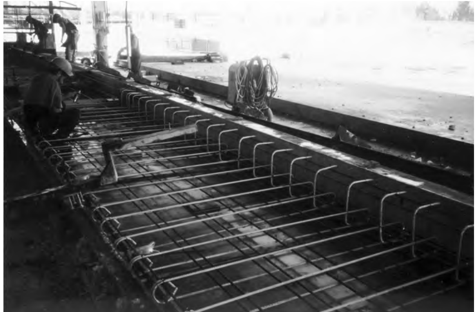
Figure 7-1 Ledged spandrel in form
