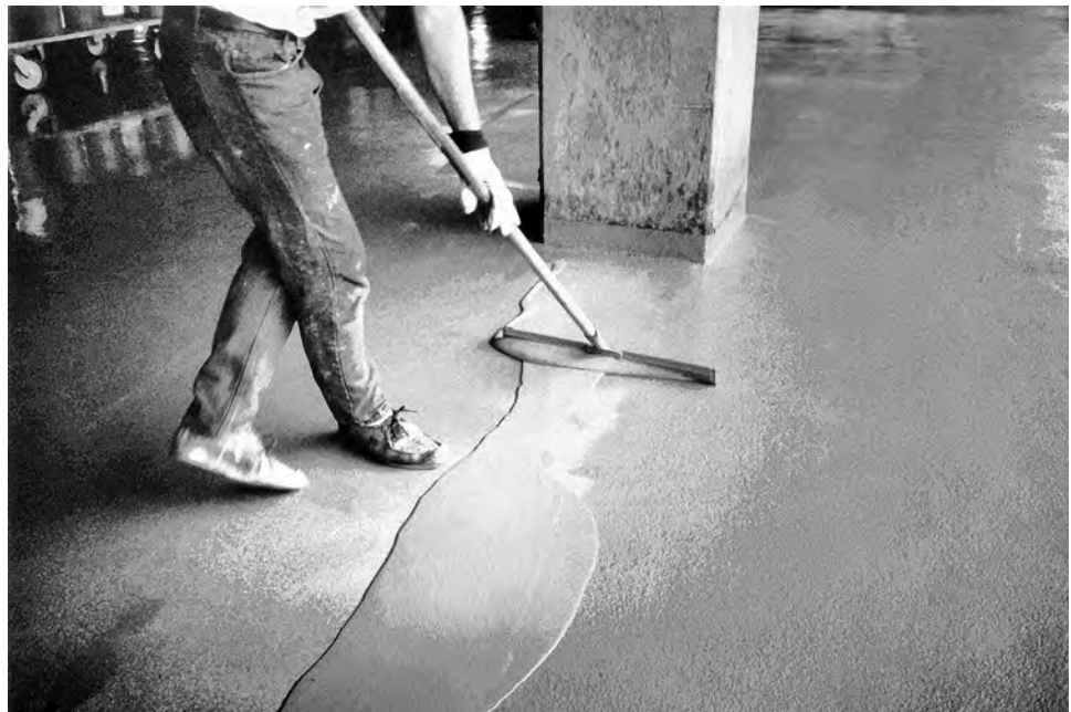
Figure 3-6 Application of Deck Membrane
