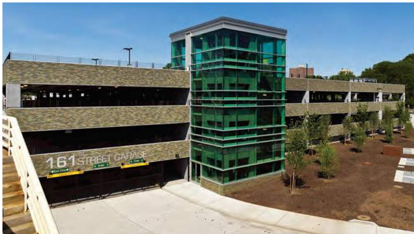
Figure 1-10. Yankee Stadium 161st Parking Garage C - New York, NY (photo courtesy of Jeffery Totaro Photography)
