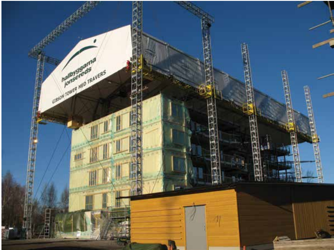
Figure 60 Use of an adjustable tent – Sweden
