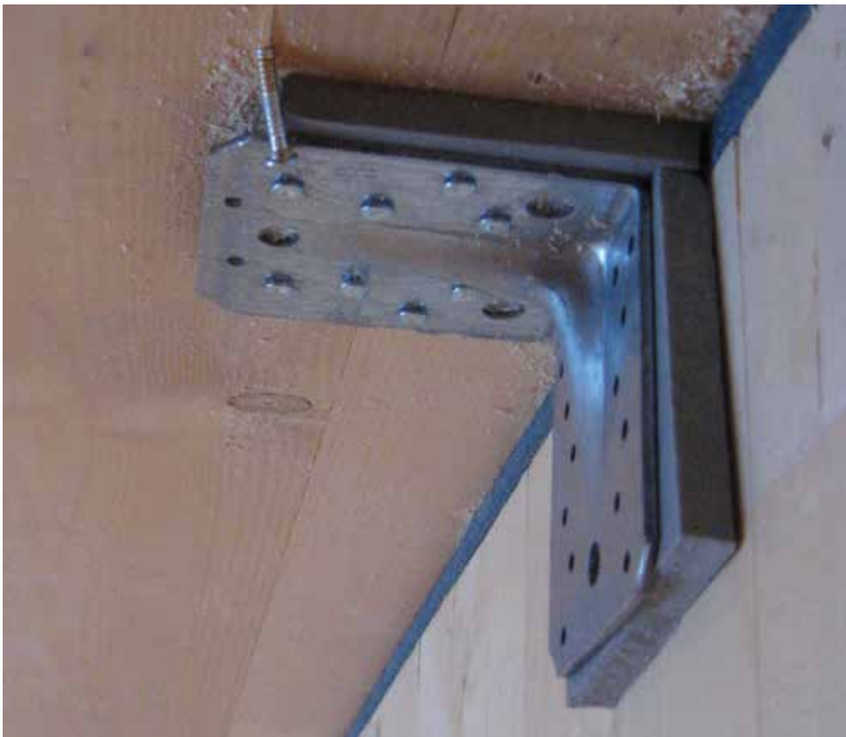
Figure 41 Sealing joint between floor, wall, and connectors
