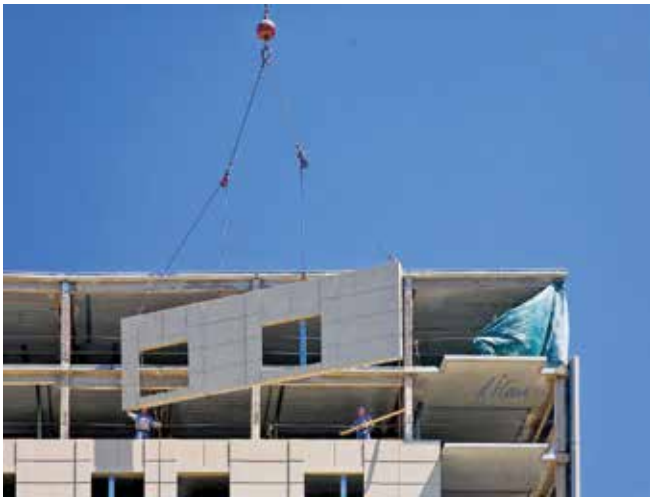
Figure 1 Lifting and handling of precast concrete elements
