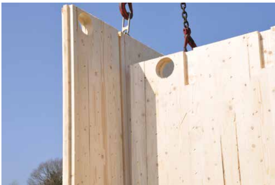
Figure 25 Screwed anchor
