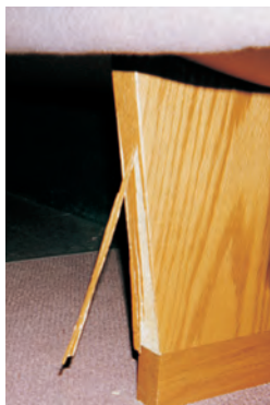
Avoid: veneer edge banded pew supports. This method is susceptible to peeling.
