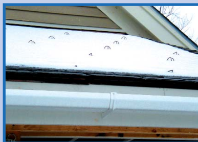
Residence, Morrisville, VT Model #70 on a slate roof.
