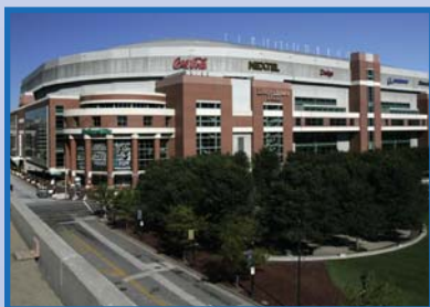
Edward Jones Dome, St. Louis, MO Model #115 on a membrane roof.
