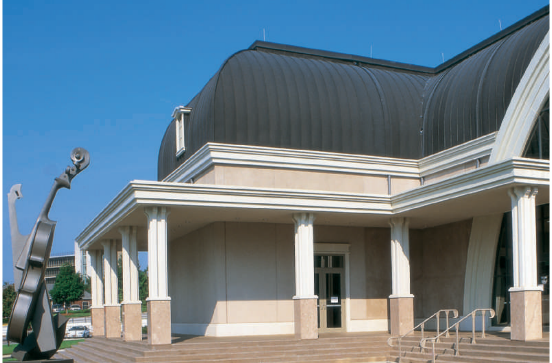
Standing seam (ANTHRA-ZINC®) Brenau Performing Arts Center, Gainesville University (USA) Architect: Lord Aeck Sargent Architecture - Contractor: Ben Hill Roofing
