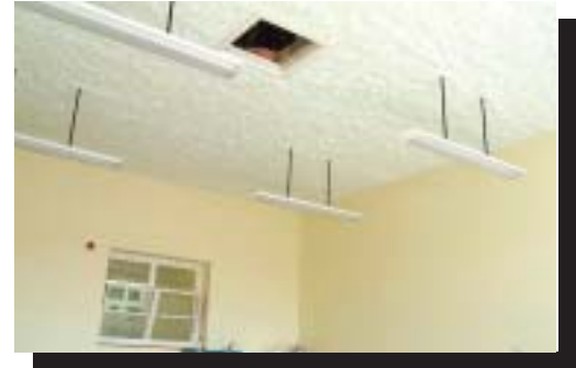
Acoustic ceiling application, School for the Deaf, London, U.K.
