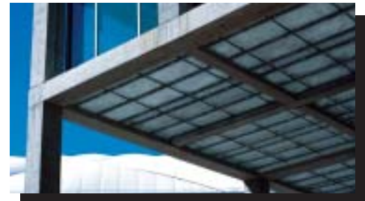
Soffit application to insulate occupied space above
