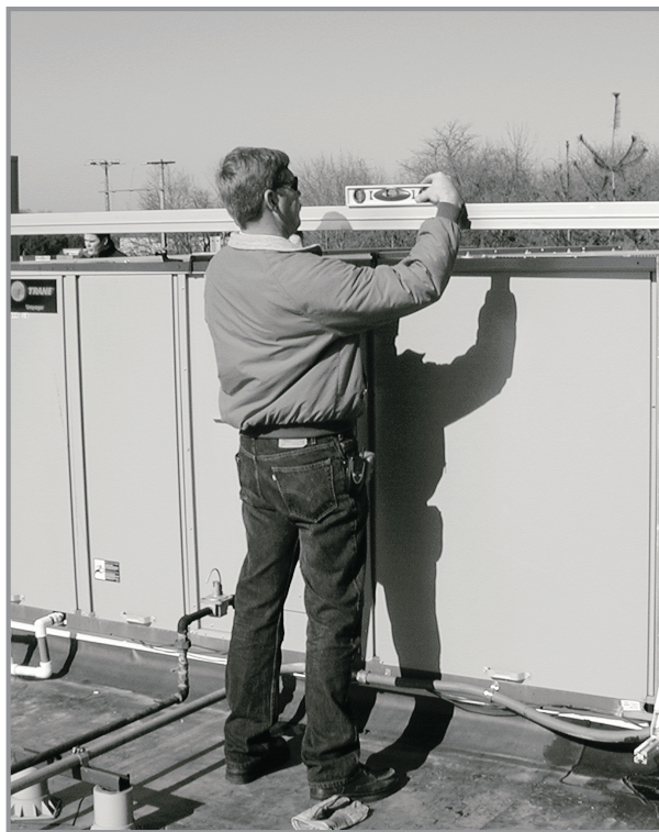
LEVELING THE COMPONENTS
