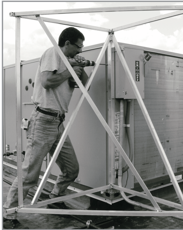
CORNER TRUSS INSTALLATION
