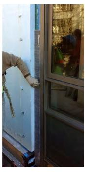
Thin-profile *Dow Corning*® HPI-1000 Building Insulation Blanket can be cut to fit and easily installed in tight areas such as window openings to prevent thermal bridging.
