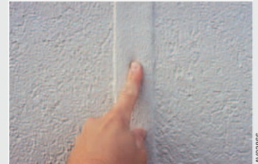
EIFS joint restored using Dow Corning® 123 Silicone Seal
