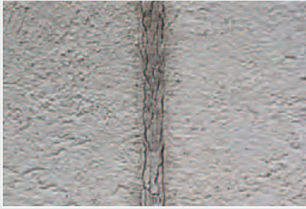
Failed urethane sealant in EIFS joint
