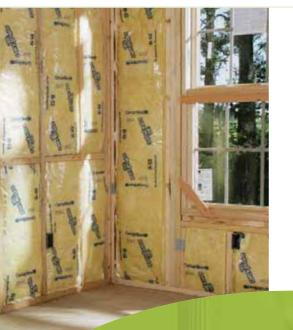
CertainTeed insulation products improve building energy efficiency and reduce building energy consumption for the life of the structure. As a result, they help conserve nonrenewable energy sources, decrease dependence on foreign oil and lower greenhouse gas emissions. In addition, the recycled content of CertainTeed fiber glass insulation meets the EPA Recovered Material Guideline for fiber glass products, 30-40% consisting of pre-consumer and post-consumer glass cullet.
