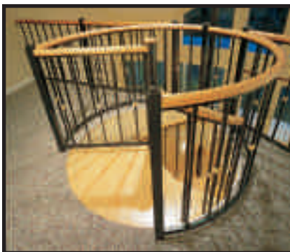
270° circular guard rail with 2" oak handrail and 5/8" square balusters with collar
