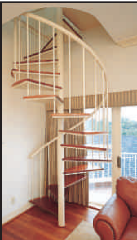
64S 2" Rd. handrail, 3/4" Rd. balusters, # 140 mahogany treads
