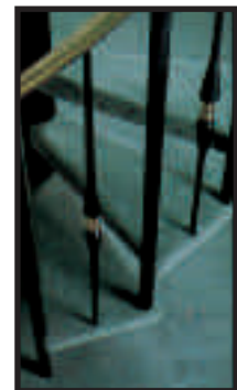
52S w/opt. 220 bronze handrail w/328 center baluster
