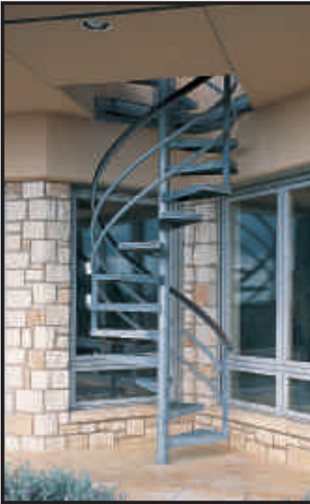
48S 3 line rail, radial grate treads, galvanized
