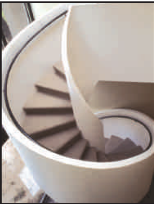
Custom curve 6'6" diameter w/oak treads and closed risers, dry wall by others
