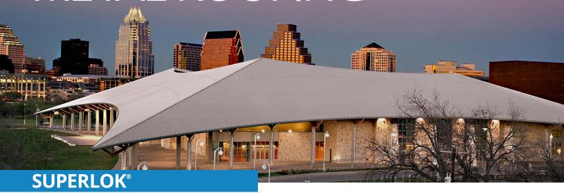
SuperLok® is a mechanically field-seamed, vertical leg standing seam roof system that combines a 2" tall slim rib with exceptional uplift resistance. It is available in both 12-inch and 16-inch widths. SuperLok® has been designed to withstand the most rigorous weather conditions. SuperLok® can be installed directly over purlins or bar joists. SuperLok® does not require a solid substructure for support.
