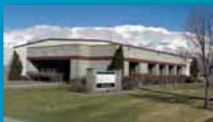
INTERSTATE GRATINGS, UT ▲
