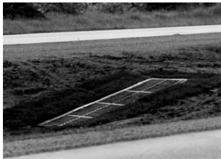
MEDIAN DRAIN AND FREEWAY DRAINAGE
