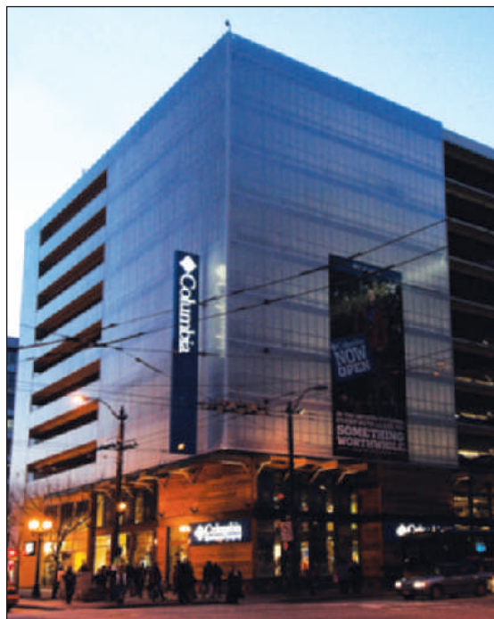
ID 27205 - Third & Pine Parking Garage, Seattle WA Architect: Sienna Architecture, Portland, OR CPI provided 24,000 SF of Pentaglas® 10 finished with Ice White Matte glazing to clad an existing 8-story open parking garage. The glazing system and use of reversed battens created an aesthetically pleasing flush look to compliment the heart of downtown Seattle.
