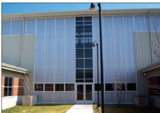
ID 10851 - Nashua High School, Nashua, NH Architect: Lavelle Bresinger Architects, Manchester, NH CPI provided 6,400 SF of Quadwall® LiteWall™ panelized in 6' modules.
