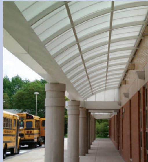
ID 17988 - Speed School, Chicago Heights, IL Architect: Detella Planera Paukner Architects, Olympia Fields, IL CPI self-supporting drop-off canopy.
