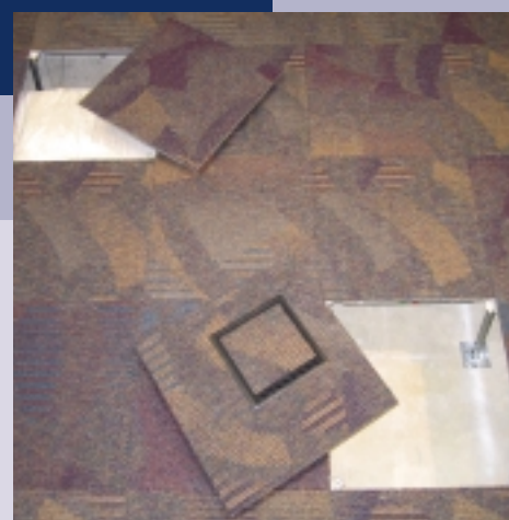
Step 3: Switch the service panel with the solid panel...
