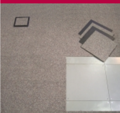
Step 1: Remove four 18"x18" carpet tiles to expose one panel...
