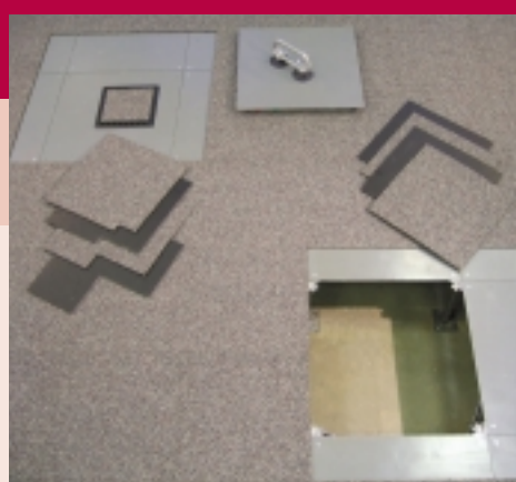
Step 2: Remove four cut carpet tiles from around service box...
