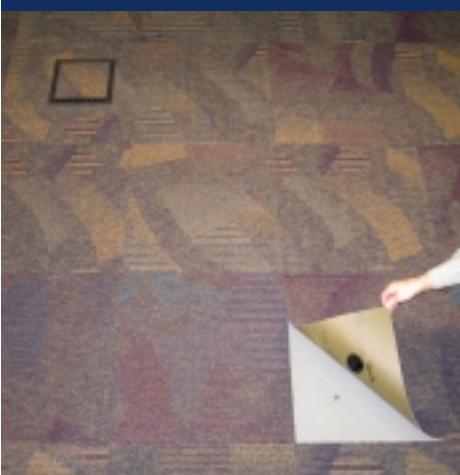
Step 1: Remove one PosiTile® carpet to expose one panel...
