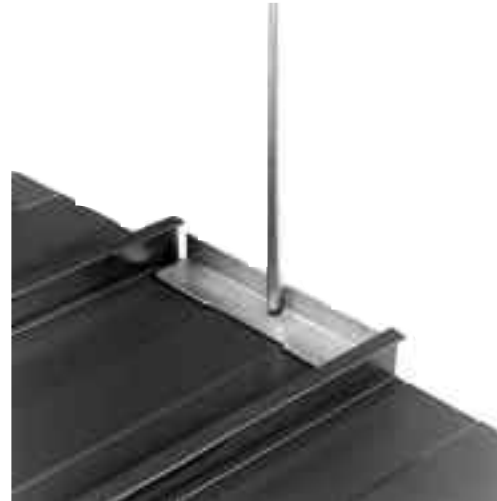
Figure 16. Panned End Panel Assembly.
