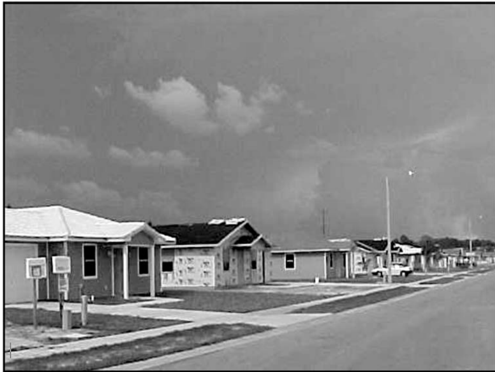
Figure 2. Picture showing the Habitat for Humanity test homes in Ft. Myers, Florida.
