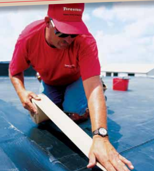
The Firestone QuickSeam Tape Seam System is the most advanced method of field seaming RubberGard EPDM membrane available in the industry.
