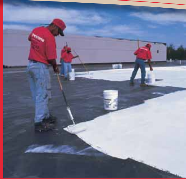
Firestone's Acryli Top™ coating helps extend an EPDM roof's service life.
