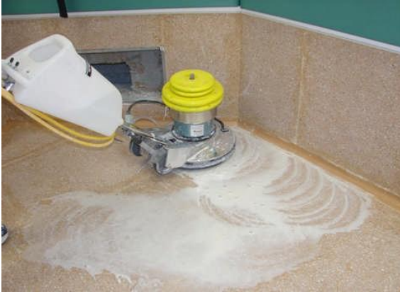
Wet-polishing procedure to remove residue and eliminate lippage.
