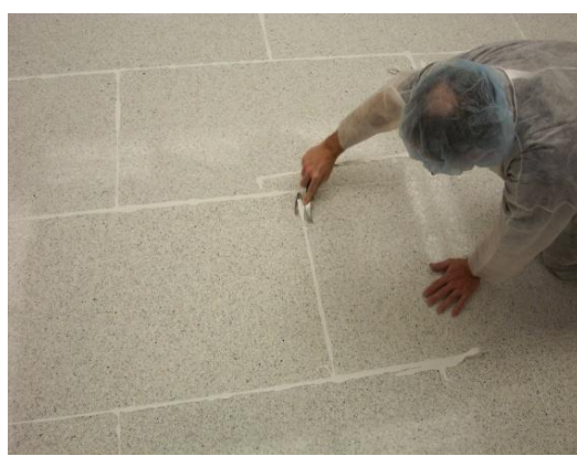
Remove excess FUSION™
