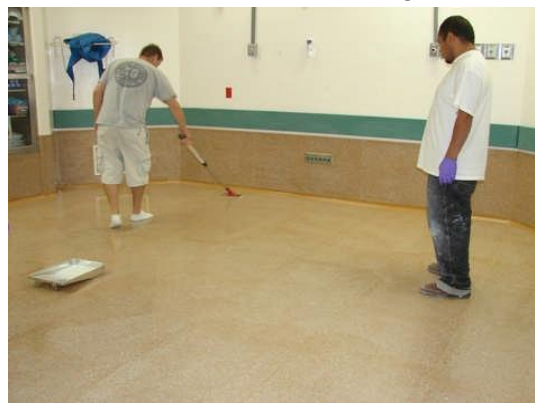
Apply cleaning solution with a mop and bucket, scrub, and remove remaining solution with wet-vac.
