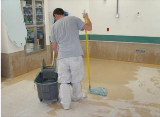
Apply cleaning solution with a mop and bucket, scrub, and remove remaining solution with wet-vac.
