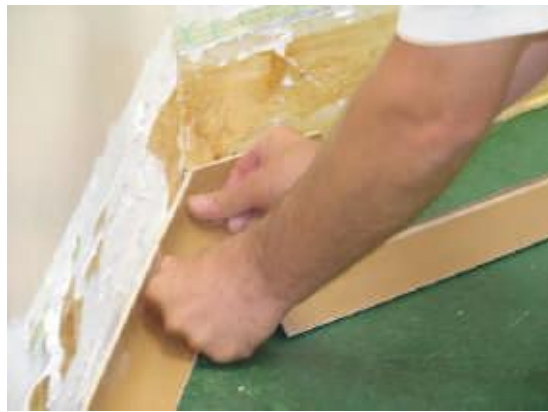
Secure base into position with adhesive
