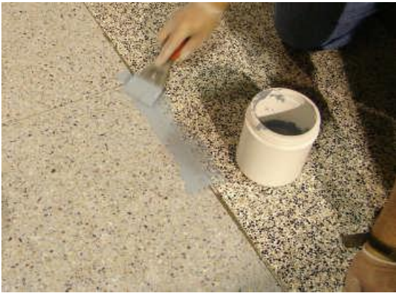
Apply FUSION™ to joints
