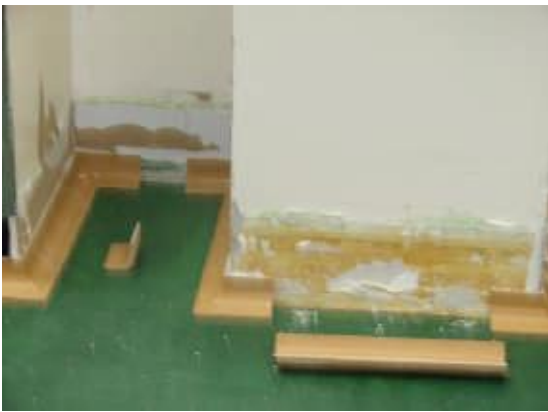
Cut sanitary base to fit
