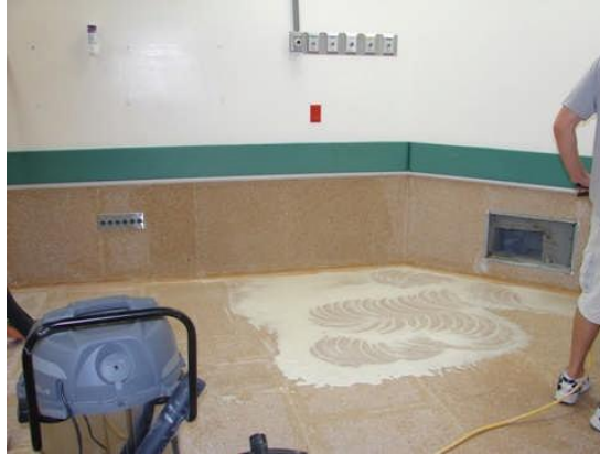
Wet-polishing procedure to remove residue and eliminate lippage.
