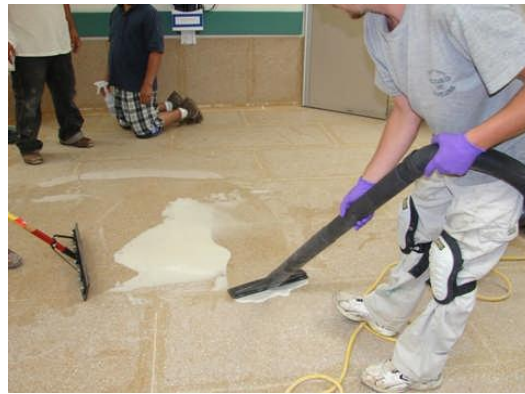
Apply cleaning solution with a mop and bucket, scrub, and remove remaining solution with wet-vac.
