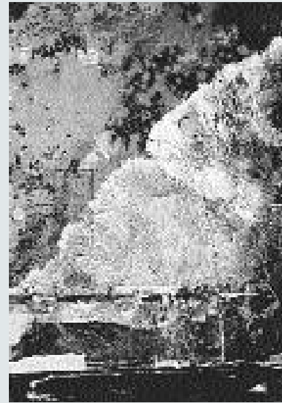
Mycelium of a wood-rotting fungus growing under the siding of a house. The mycelium is essentially the digestive organ of the fungus, secreting enzymes designed to digest the substrate (such as a cellulose-based building material) so that the dissolved nutrients can be absorbed.
