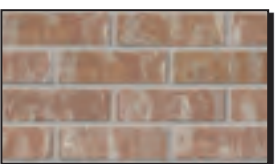
Ironstone Denton Plant
