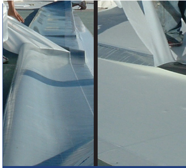
2. Remove Release Films And Adhere Membrane
