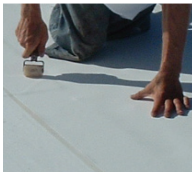
3. Roll Edges, Seams, & Field Of Roof
