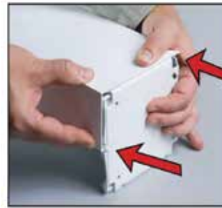
Hook top lip of fascia onto bracket
