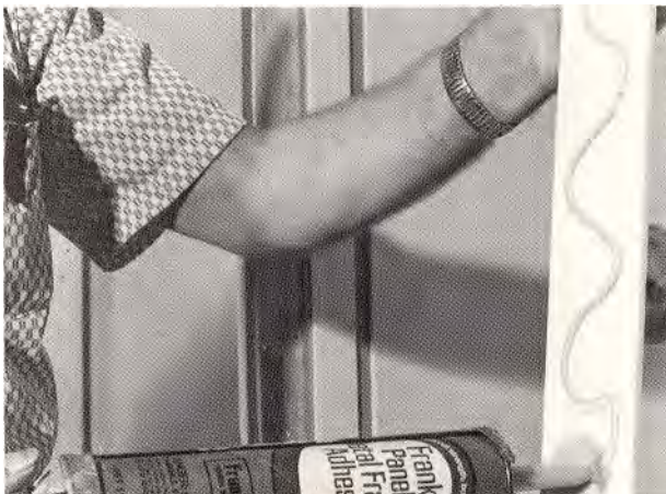
Install casing strips
