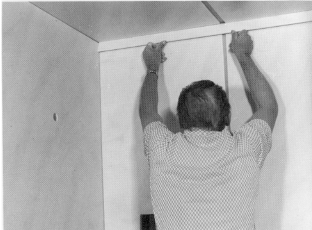
Install ceiling trim
