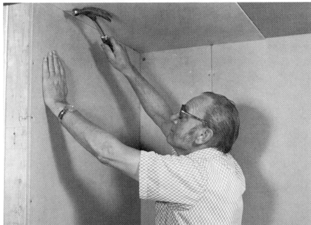
Cut and install ceiling panels
