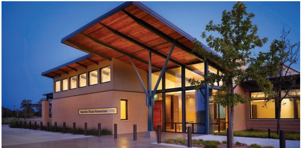
Greater Texas Foundation, Bryan Texas Photo courtesy of Page
