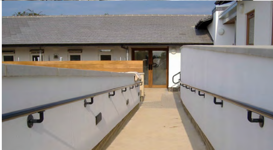
Right: ADA Compliant Railing for Access Ramps
