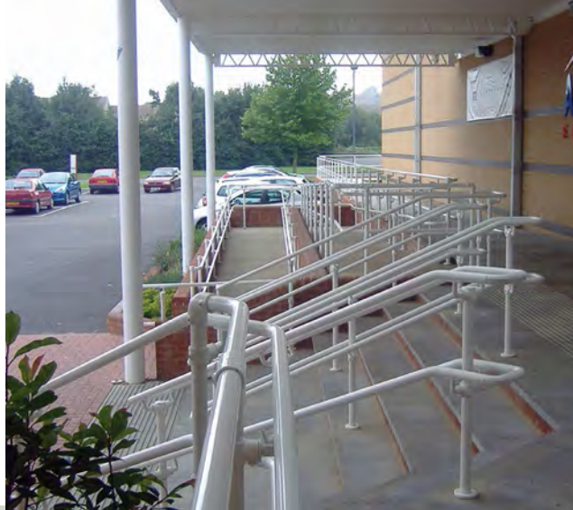
Right: ADA Compliant Railing for Public Access
