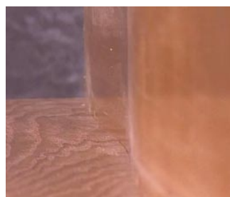
STEP 3 There is no need to caulk when you achieve a precise fit.
