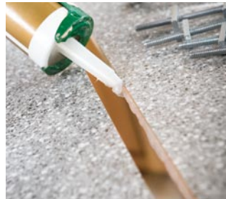
STEP 1 Apply silicone sealant.
