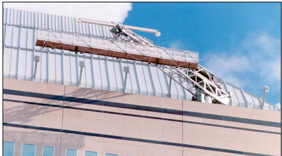
Roof car with traction hoists and wire winders on roof car. Platform is 40'-0" (12.2 m) long.
