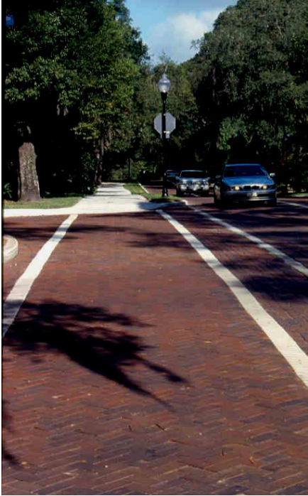
New Traffic Calming Clay Pavers
