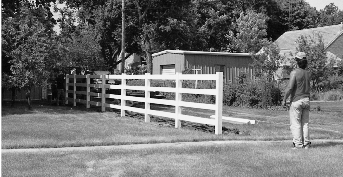
Aligning the fully assembled fence before final tamping.
