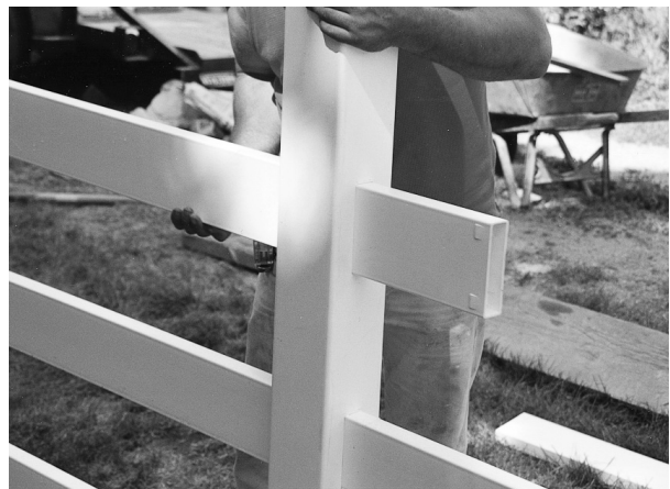
Rails are threaded through the pre-routed posts.
