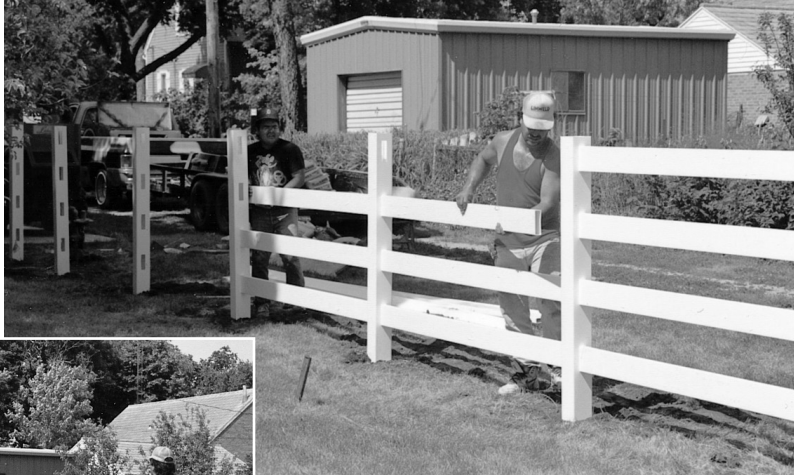
Aligning the fully assembled fence before final tamping.
