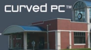
Mechanically seamed in the field, these 1" or 1-1/2" high curved standing seam panels provide weathertightness and durability for your curved panel design projects.
