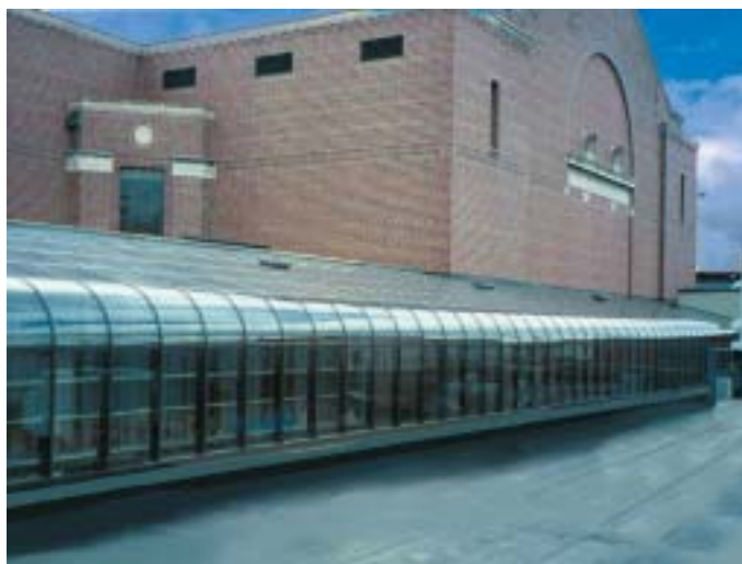
Ohio State University Walkway • Ohio
