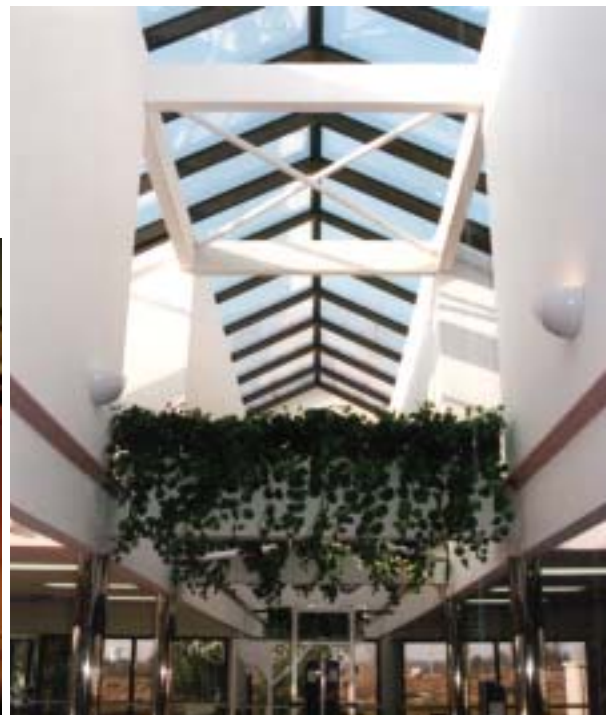
Skylight • Community Fitness Center, OH
