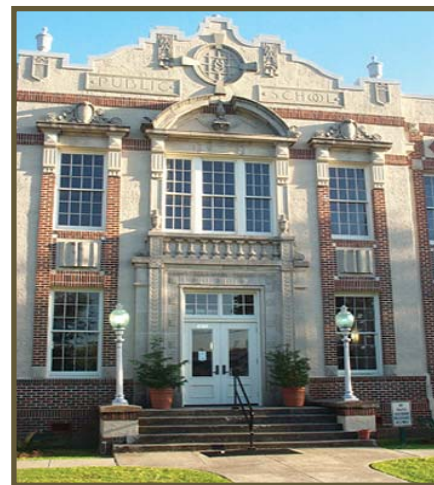
Historic Schoolhouse 2nd Floor Sound Studios.
