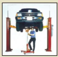
Mohawk's Patented hydraulic equalization eliminate floor plates and overhead obstruction, giving you a clear floor work space for complete access under any vehicle.
