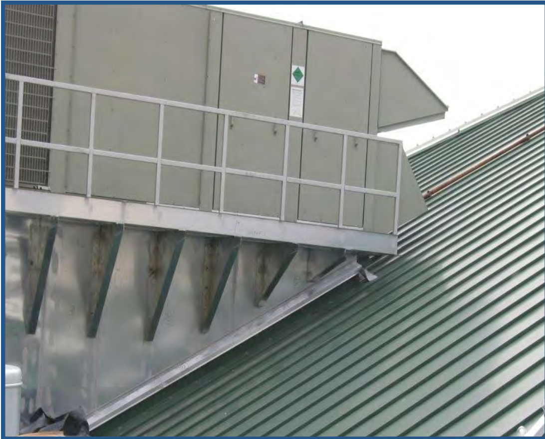
Metal Building Catwalk Curb
