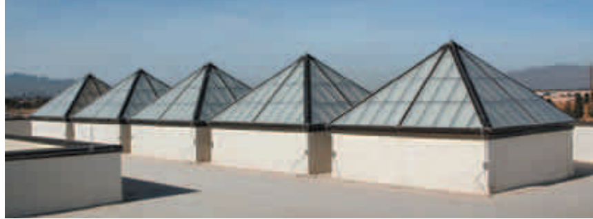
Headworks Digester Plant - Las Vegas, NV HDR Engineering
