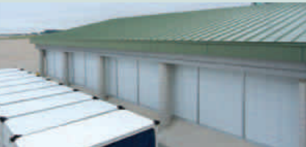
Lambert International Airport - St. Louis, MO Burns and McDonnell Architects
