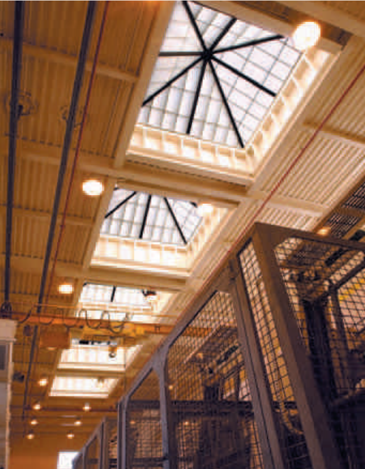
Headworks Digester Plant - Las Vegas, NV HDR Engineering
