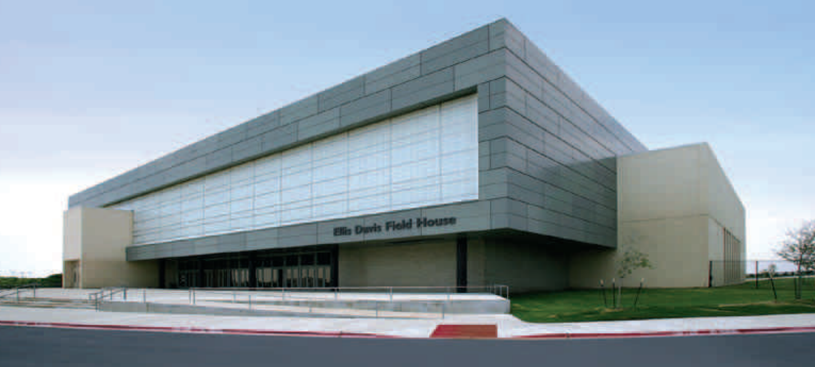
Ellis Davis Field House - Dallas, TX HKS, Inc.
