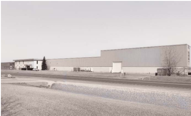
124th Street Facility in Wauwatosa, Wisconsin
