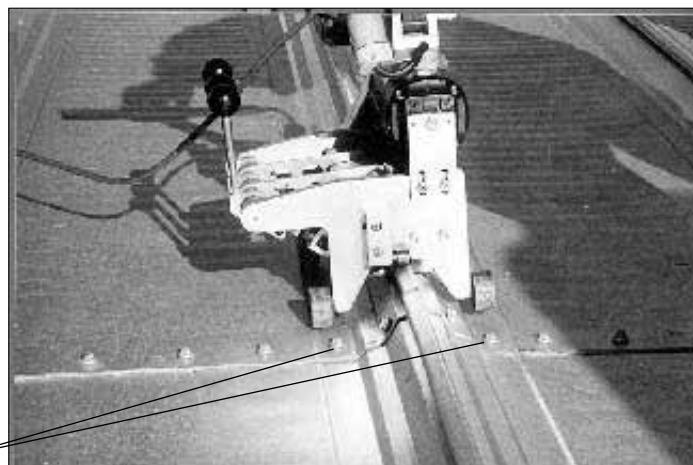
Photo 3B Electric Seaming near endlap
