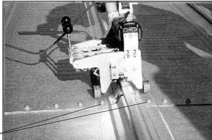
Photo 3B Electric Seaming at Endlap
