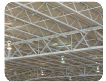
Continuous Truss with WideBay
