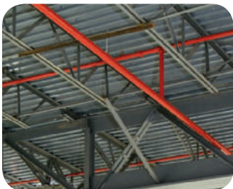
Continuous Truss with Transbay
