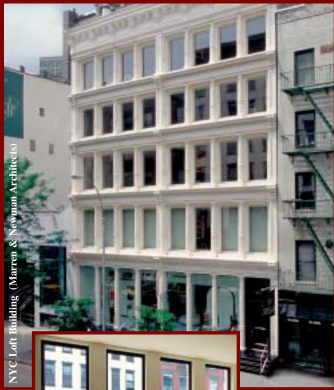
Custom designed Megawood+Bronze™ windows are a unique replacement for the 12' tall original bronze double hung windows. A fixed over tilt-turn window with offsetting glass planes met the stringent Landmark's historical requirements.
