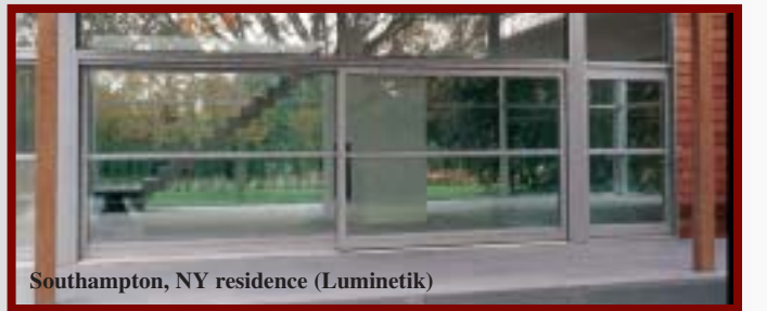
Huge operable windows and doors with thin framing are standard Megawood™ features that accentuate this modern design. Extra-wide swing doors and 11' wide lifting-sliding doors blend seamlessly with fixed, tilt-turn and hopper windows throughout all elevations of this residence.
