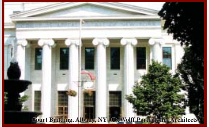
Custom designed Megawood+Bronze™ windows are a unique replacement for the 12' tall original bronze double hung windows. A fixed over tilt-turn window with offsetting glass planes met the stringent Landmark's historical requirements.
