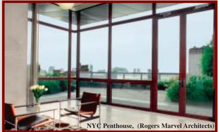
Fixed windows, hoppers and 10' tall french doors combine to form a stunning Megawood+Aluminum™ penthouse window-wall with slender mullions and a butt-glazed corner to make the most of the Hudson River and city views. Narrow hardwood interior framing was finished with a rich mahogany stain.
